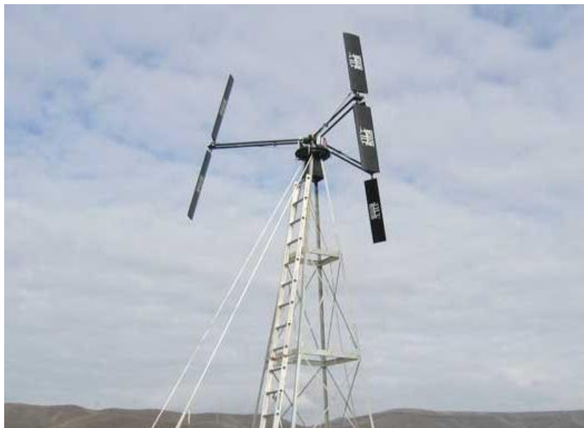
Figure 7: Installation of a BlackHawk TR-10 VAWT [21]
